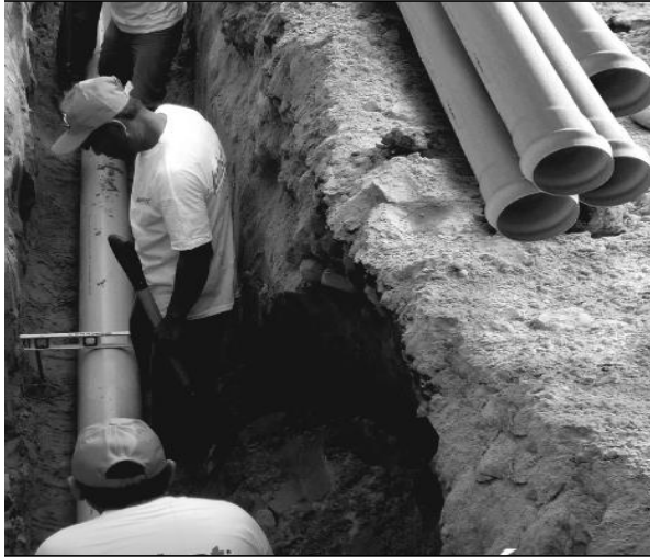
Figure 2. Water networks construction in El Pedregal.
